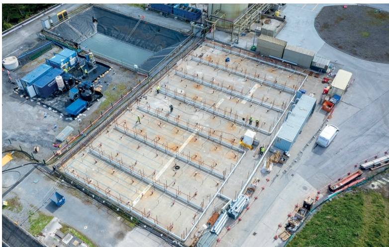
An aerial view of AEC 2 being remediated using in situ thermal treatment
