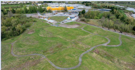
The landfill prior to the commencement of preparatory works.
