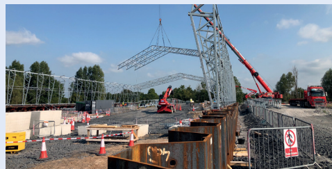
September 2024: The first enclosure being secured onto the sheet piles.
