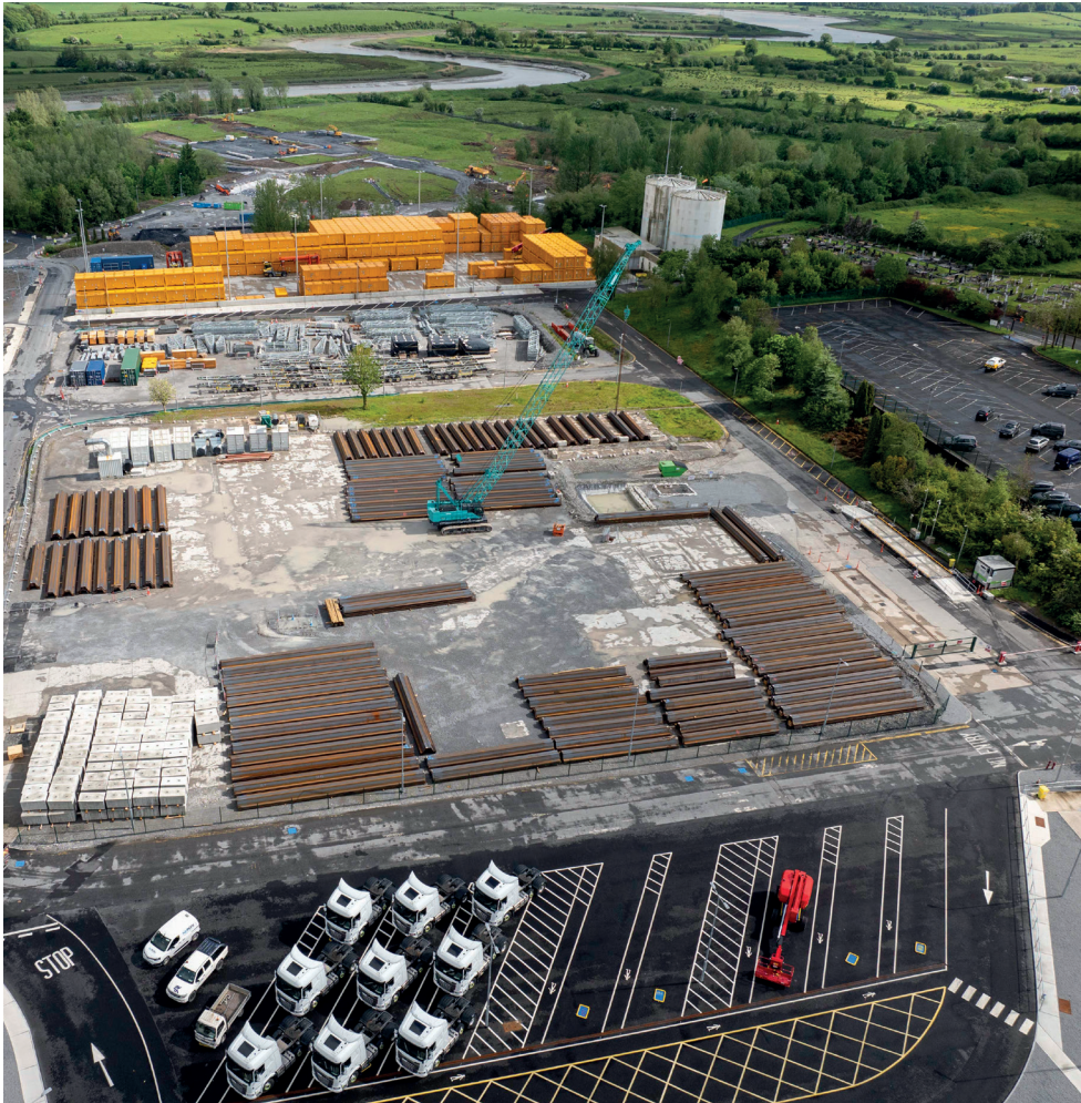
April 2024: The steel sheet piles arriving to-site.
