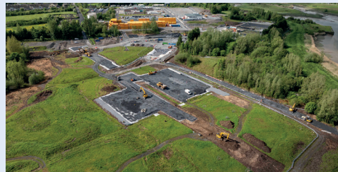
May 2024: Enabling works underway to facilitate sheet piling.
