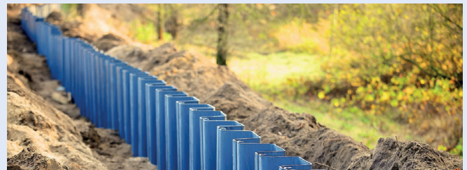
Sheet piling to be used to support the installation of the enclosures. (Simulation)
