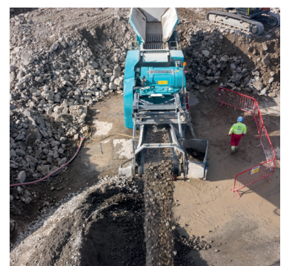
30,000 tonnes of concrete emanating from the 'Demolition' phase have been crushed on-site.
