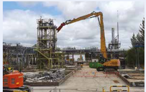
Machinery used during the 'Clean to Shell' and 'Demolition' phases - Brokk demolition robot used to remove equipment from buildings (left) and high-reach machine being used during demolition (right).
